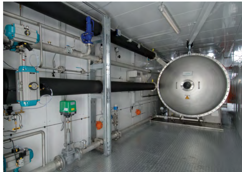
Ozone generator and pipework installed in container
