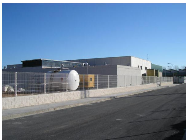
Figure 1: Falconera Water Treatment Plant
