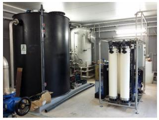
Figure 2: Raw water tanks (left) beside the aquasource Z-XS unit (right)
